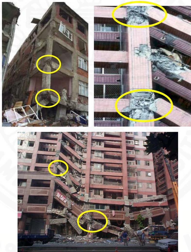
Fig. 1.1 Failure of beam-column joint may lead to catastrophic collapse of the entire building.
